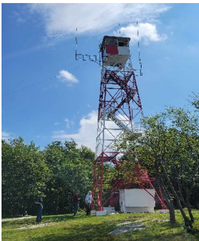
Culvers Fire Tower
